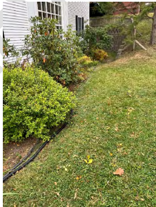
Photo 14 – Outlet of exterior sump pump
