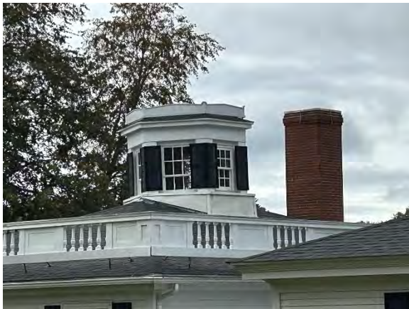
Chimney & Cupola at the Tisdale House
