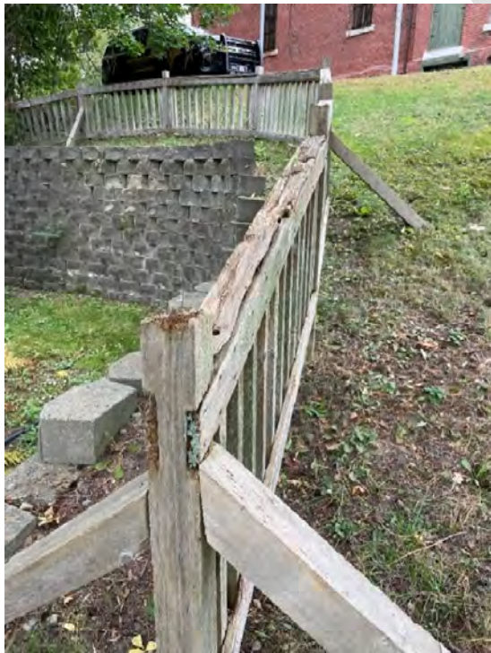
Photo 27 – Top of wall fencing, typ
