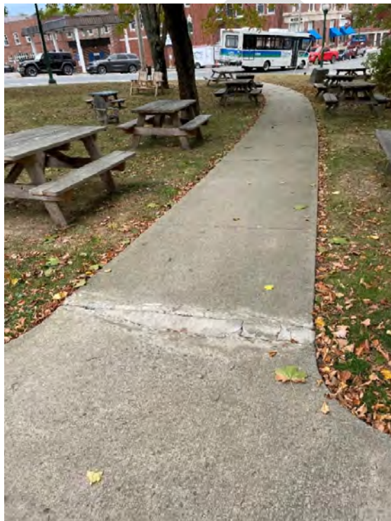
Photo 5 – Concrete sidewalks from State Street
