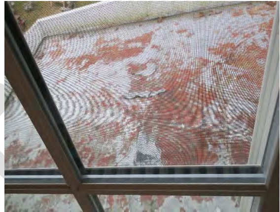
Tin Roof at the Tisdale House Entry
