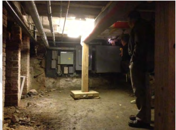
Dirt Basement at the Tisdale House
