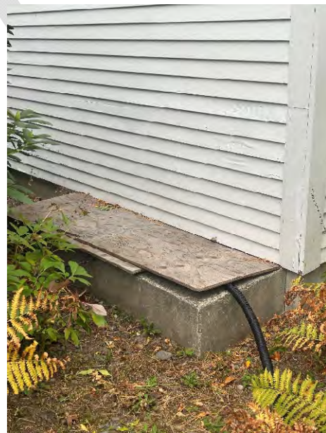
Exterior Window Well
