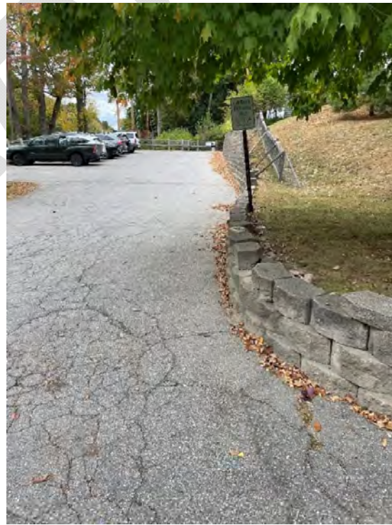
Photo 18 – Asphalt paved parking lot
