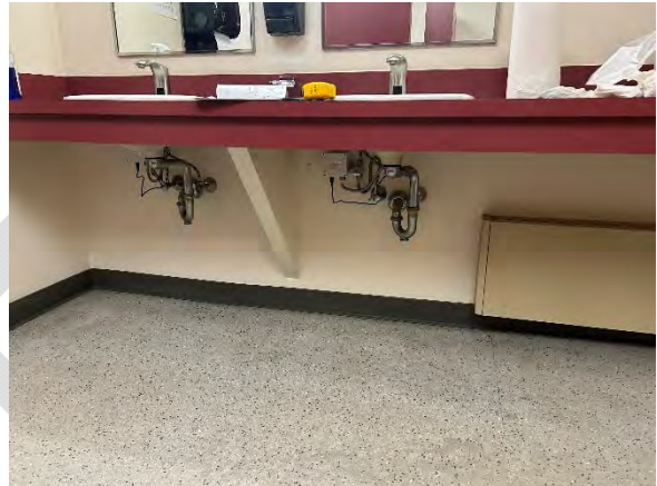
Exposed Sink Pipes at the New Addition
