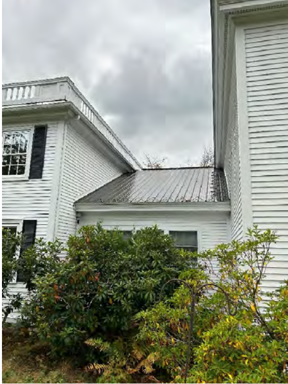
Standing Seam Roof at the Connector
