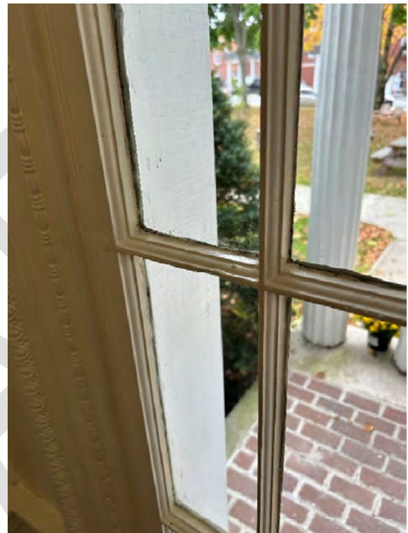
Single-Pane Sidelight at the Entry Door
