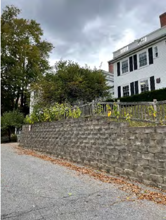
Photo 21 – Retaining, east side of parking
