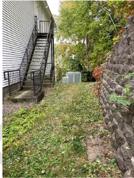
Photo 12 – Area of poor drainage near fire escapes
