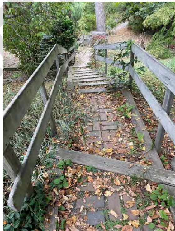
Photo 6 – Brick/timber path to River Trail
