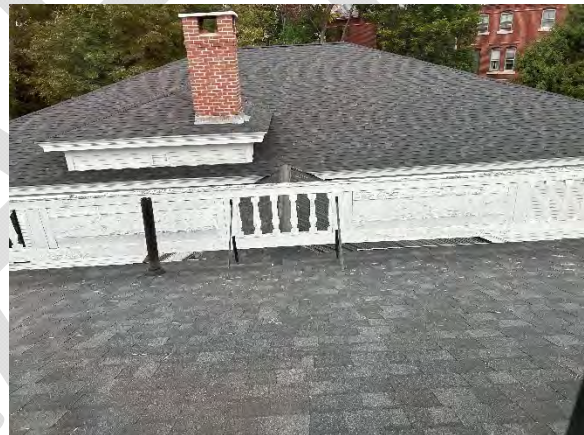
Chimney & Penthouse at the New Addition
