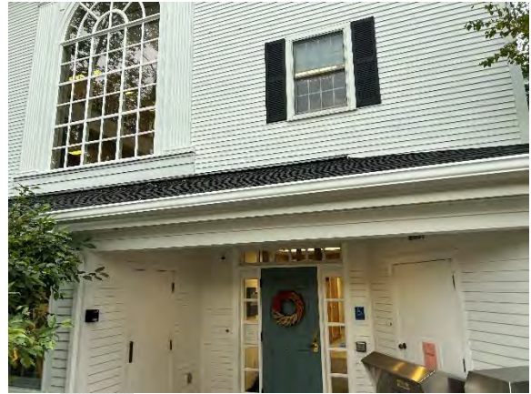
Windows & Doors at the New Addition
