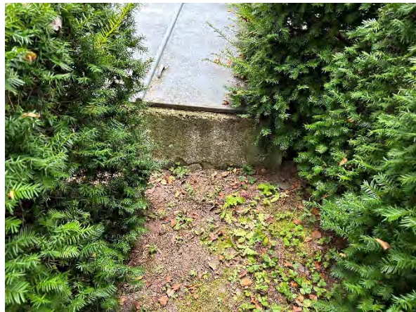
Steel Bulkhead at the Connector
