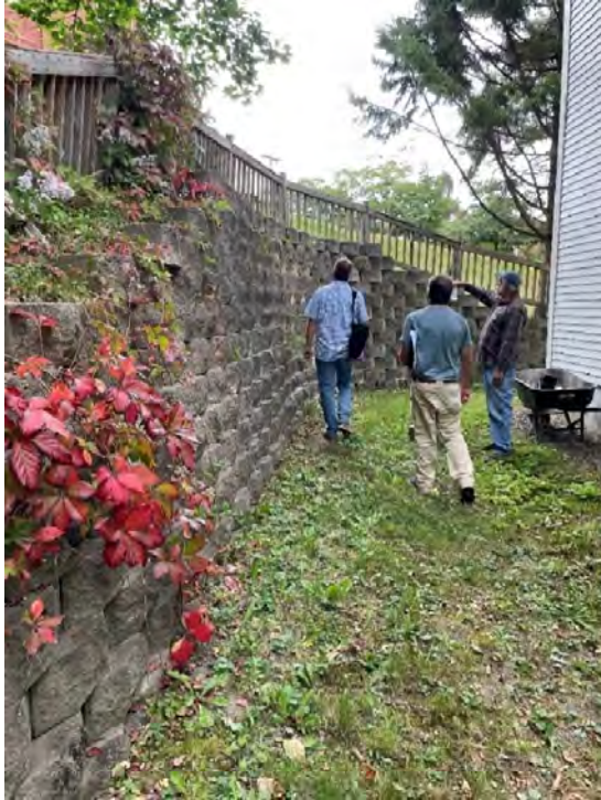
Photo 11 – Area of poor drainage near fire escapes
