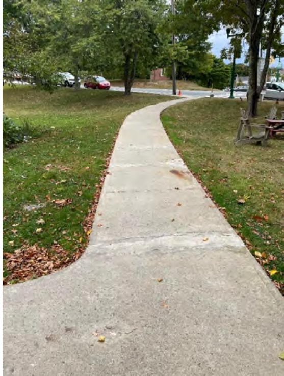
Photo 3 – Concrete sidewalks from State Street
