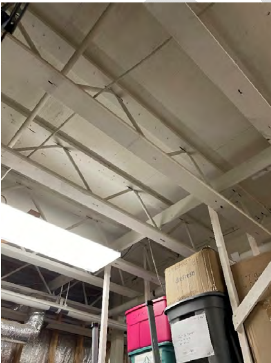
Photo 3 – First floor framing in addition, from lower level
