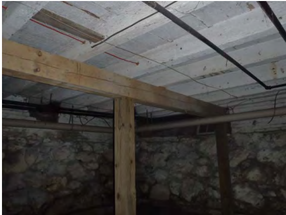
First Floor Framing at the Tisdale House
