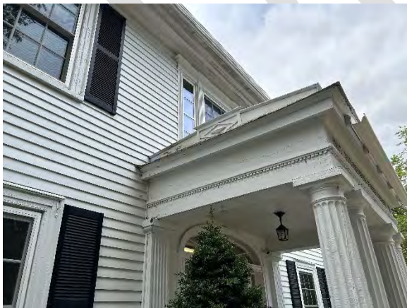
Siding & Trim at the Tisdale House
