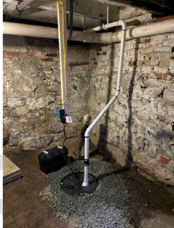
Photo 2 – grouted stone and brick foundation walls, sump pump system
