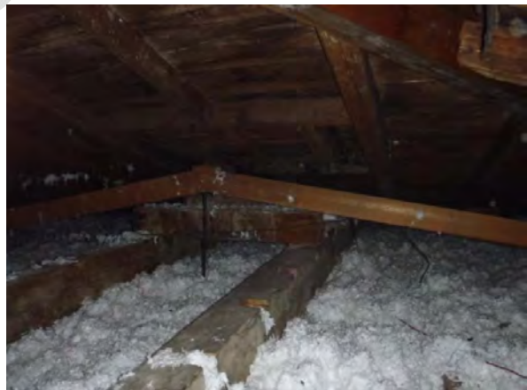
Attic Insulation at the Tisdale House
