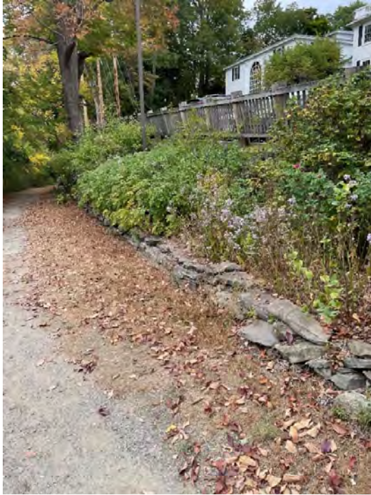
Photo 25 – Retaining, west side of parking lot
