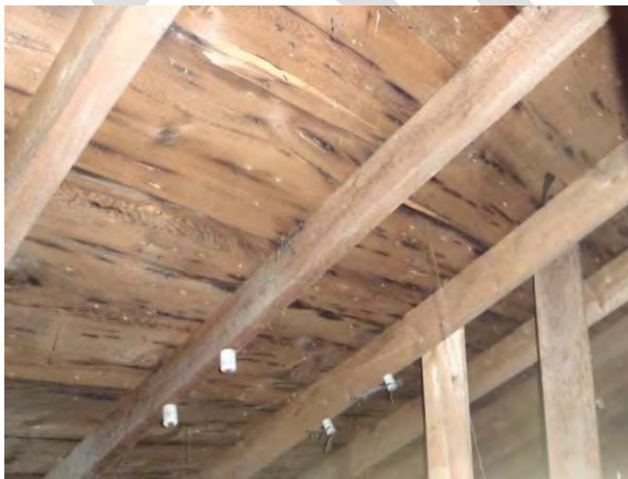
Roof Framing at the Tisdale House
