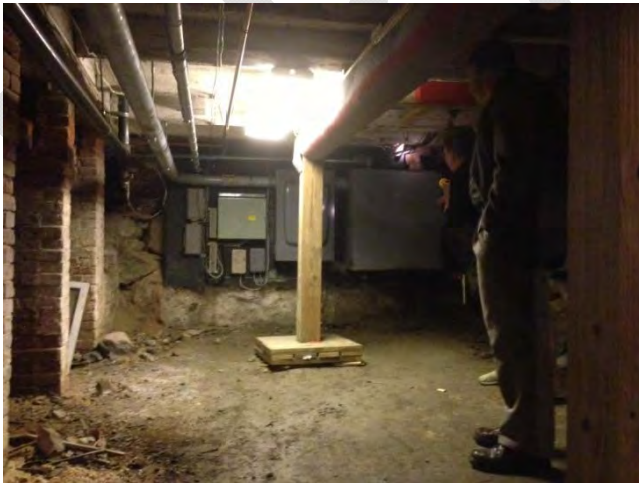
Dirt Basement Floor
