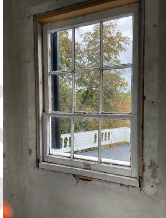
Photo 14 – Interior of cupola, window access to roof
