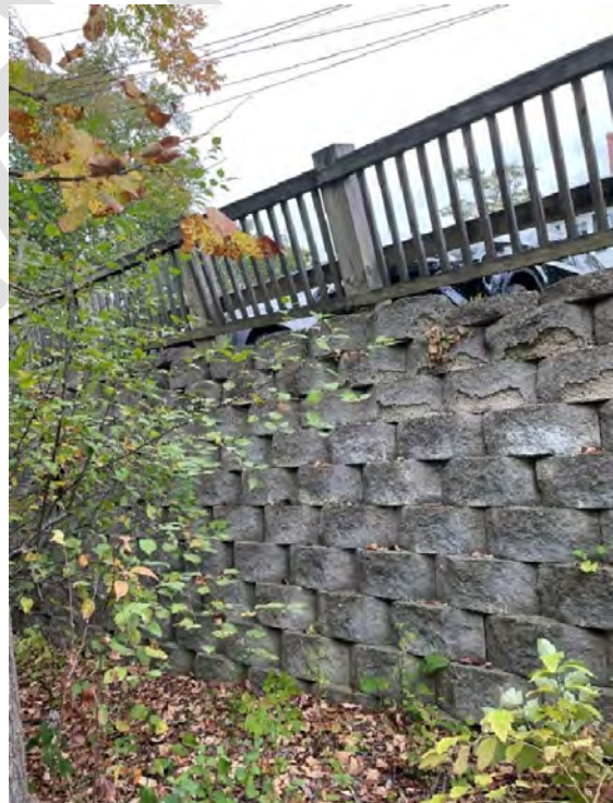
Photo 24 – Retaining, west side of parking lot
