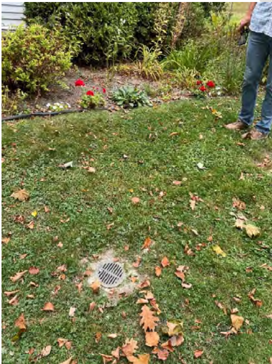
Photo 9 – Drain basin near upper main entrance
