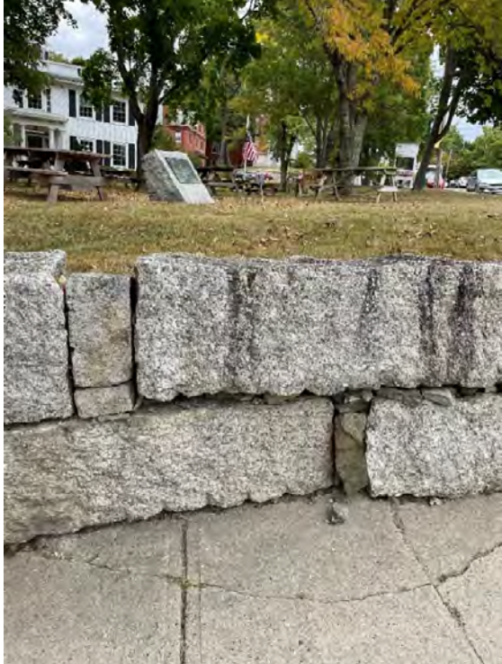
Photo 29 – Granite block wall at City sidewalk
