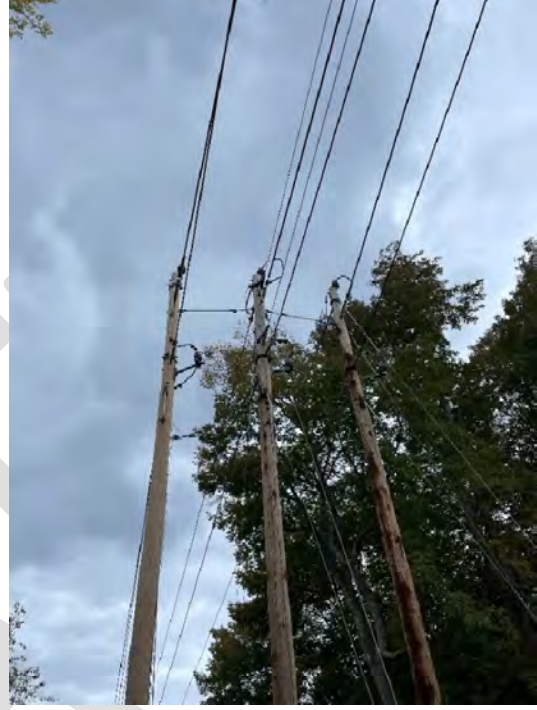
Photo 20 – Overhead hydroelectric lines
