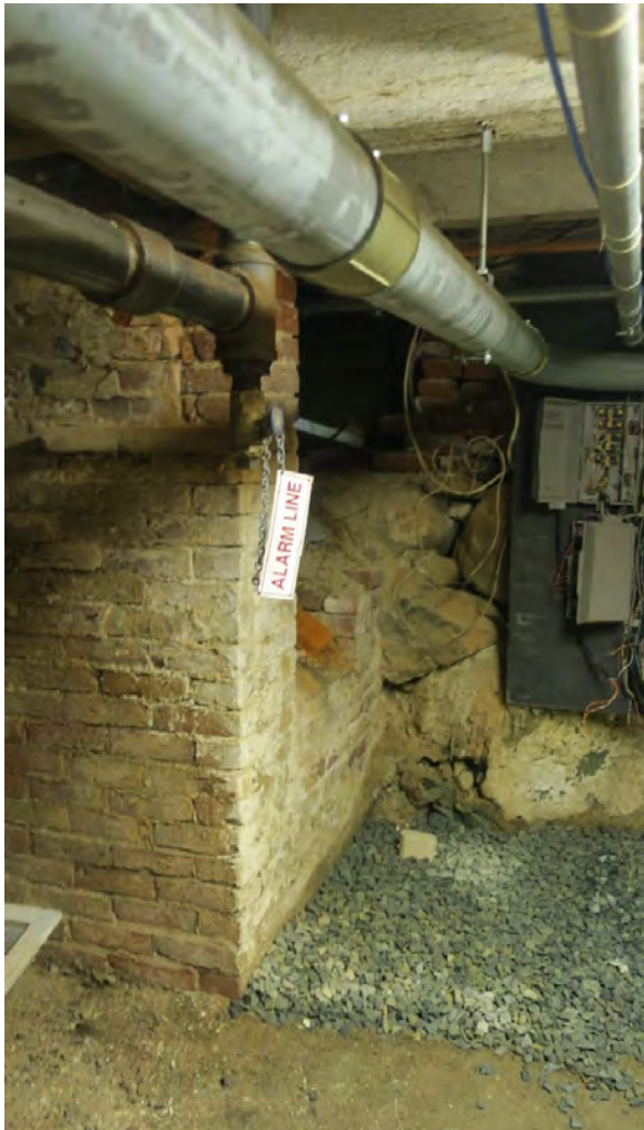
Dirt Basement Floor at the Tisdale House
