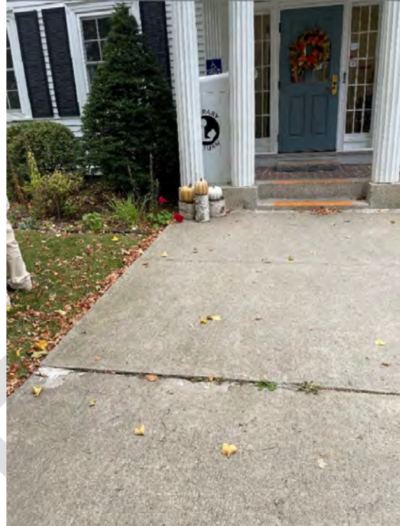
Photo 4 – Concrete sidewalk to upper main entrance
