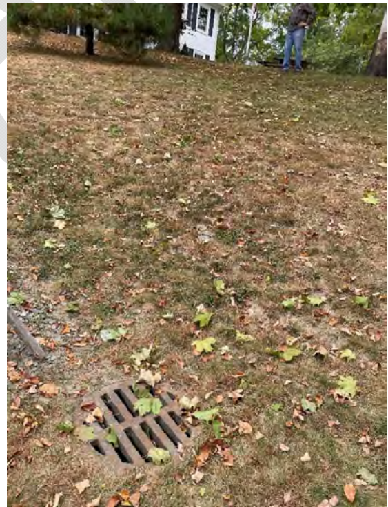
Photo 10 – Lower catch basin
